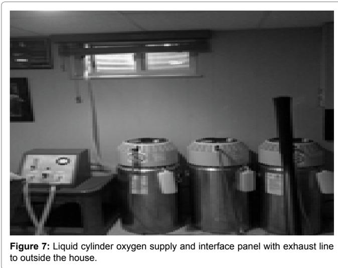
**Figure 7:** Liquid cylinder oxygen supply and interface panel with exhaust line to outside the house.
